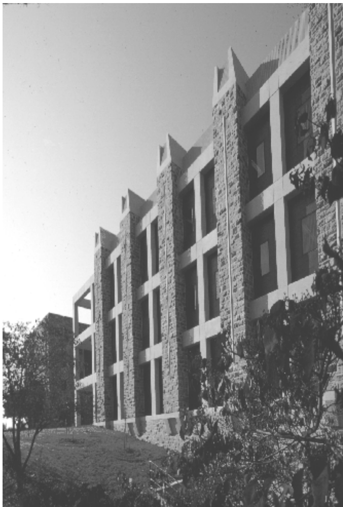
Figure 3.3 The external columns on this laboratory building, located on the campus of Virginia Polytechnic Institute & State University contain the chases for the fume hood exhaust ducts, and are located so as to serve two adjacent laboratories. The exhaust ducts are led to a common plenum and are exhausted directly upward. The laboratory module in this facility is somewhat larger than the standard module described in this chapter so as to accommodate windows. The air intakes for the facility are located to the reader's right and take advantage of the prevailing winds from that direction.
