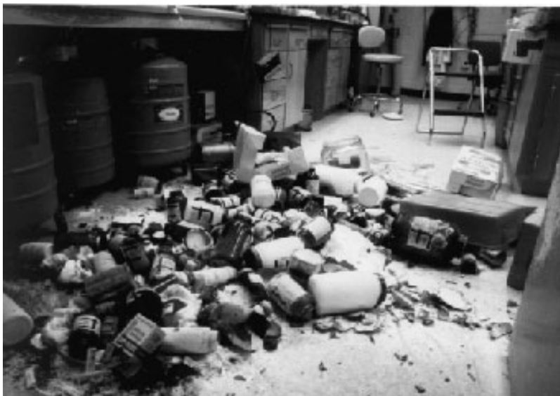
Figure 2.5 Accident due to poorly installed and weak shelving.
